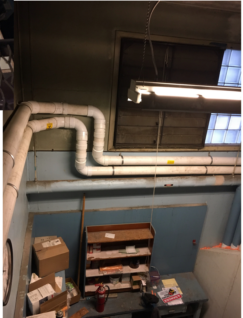
Vent pipe routing in the boiler of the facility to the fan location in the attic above.
